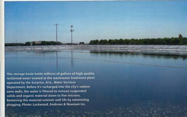
This storage basin holds millions of gallons of high-quality reclaimed water treated at the wastewater treatment plant operated by the Surprise, Ariz., Water Services Department. Before it's recharged into the city's vadose zone wells, the water is filtered to remove suspended solids and organic material down to five microns. Removing this material extends well life by minimizing plugging. Photo: Lockwood, Andrews & Newnam Inc.
